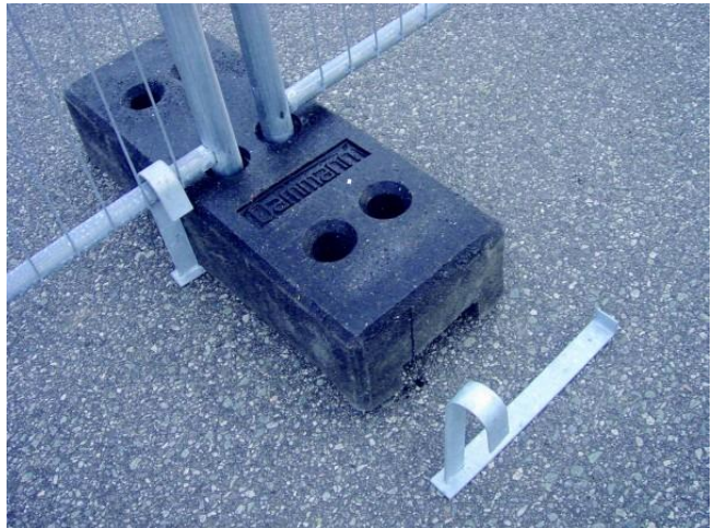
Anti-lift device for mobile fence
